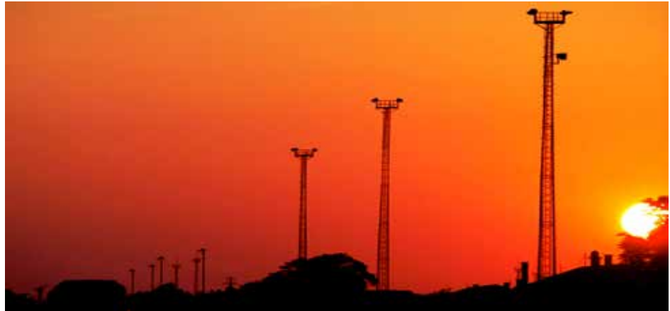
Cell towers in Kenya where mobile penetration has reached nearly 70%.
